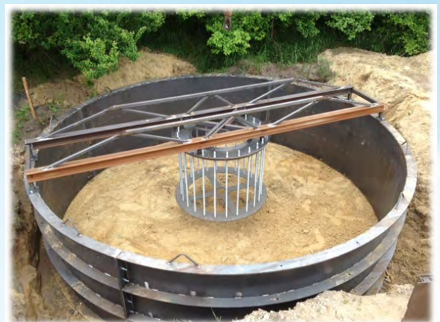
SWP 25-14 concrete foundation building process. Ringkøbing area, Denmark.
