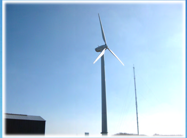
SWP 25-14 in Ringkøbing area, Denmark.
